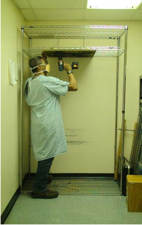
Figure 3. Picture of drilling in standing.
