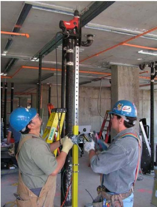
Figure 1. Inverted drill press intervention design using a rotating handle and linear gear to raise the inner (silver) column.
