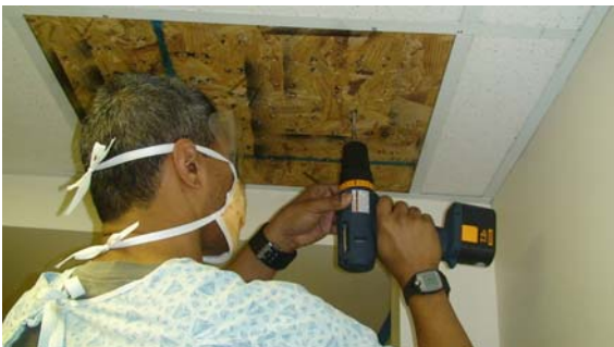
Figure 4. Picture of drilling in standing on the ladder (not shown).
